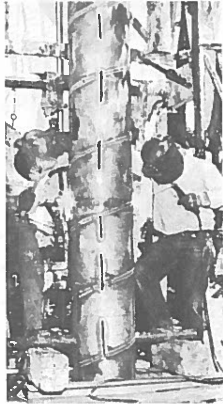
In torch-cut, slotted pipe, percent open area is low and width of slots is too large to permit developing well to sand-free condition.
